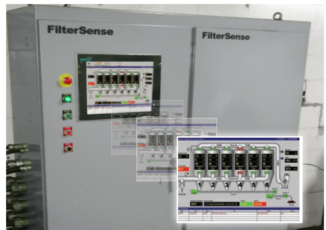
Engineered B-PAC System monitors and controls a network of multi-compartment Coke, Desulf and Casting Baghouses at a steel mill (shown left). Screenshot (lower right): shows particulate levels and damper control.
