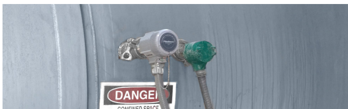
Installation of new Auburn particulate sensor (left) for filter leak detection by row.
