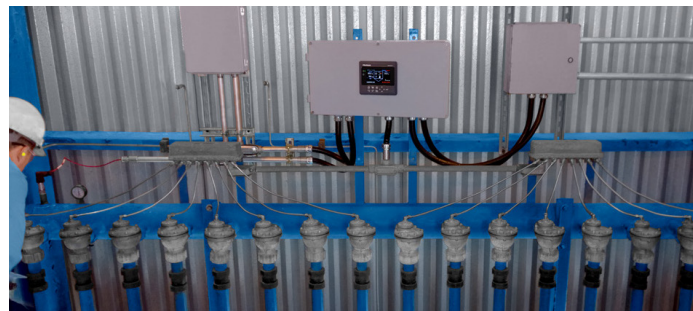
Auburn engineer inspecting B-PAC function (center) and pulse valves (below).
